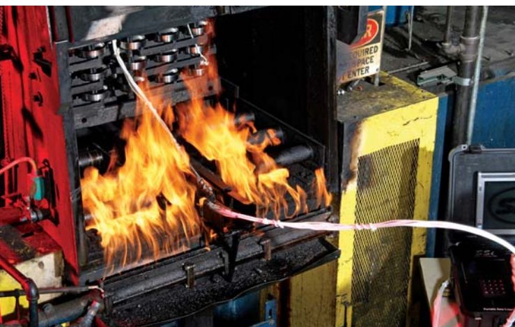
Fig. 1. Manual survey method for an integral-quench furnace (Courtesy of Super Systems, Inc.)
