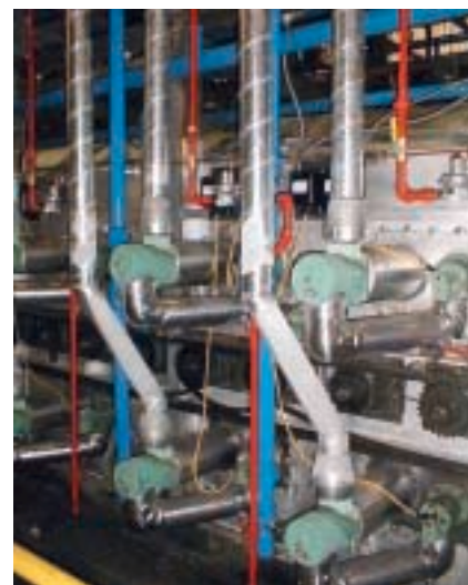
Fig 1 Modern combustion system with recuperation (Eclipse Inc. ThermThief TFB burners and Bayonet-Ultra Recuperators) installed on a continuous furnace [3]
