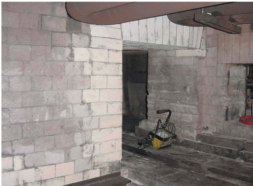
Fig. 3 — Jack-arch repair. Courtesy of Surface Combustion Inc., Maumee, Ohio.
